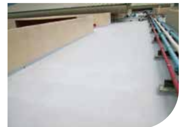
Fast-guard™ RN 500RC Primary School Roof
