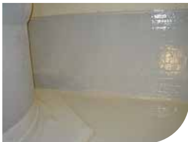
Epo-chem™ RF 500 Bund Lining
