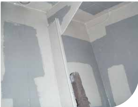
RA 500M being applied on RS 500P primed surface
