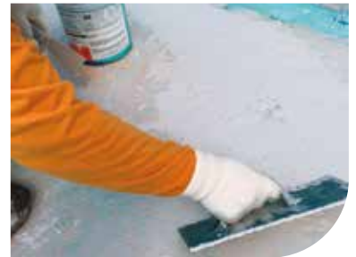
Chem-concrete™ RI 800CRS Swimming Pool Floor
