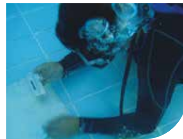
Filling swimming pool tile cracks
