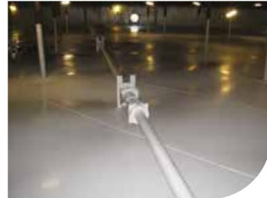
Epo-chem™ RA 500M Crude Oil Tank
