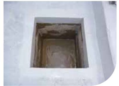
Chem-concrete™ RJ 800CRS Chemical Sump Repair
