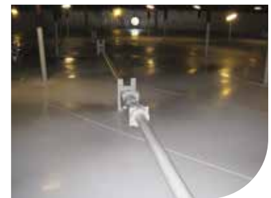
Crude Oil Tank
