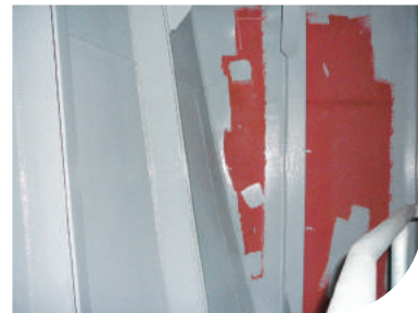
Sea Water Ballast Tank Shop-Primer Steel
