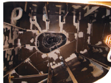
Sea Water Ballast Tank Coal-tar Epoxy Repair
