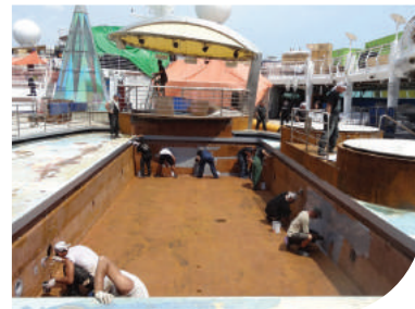
Applying Primer to Mechanically Prepared Swimming Pool
