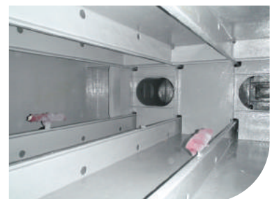
Sea Water Ballast Tank
